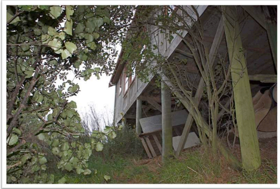
Figure 6: timber supports for the building structure
